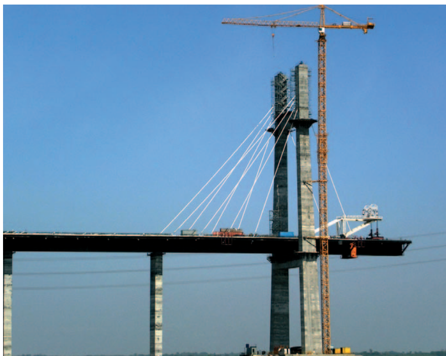
Figure 5: Free cantilever construction in progress.
