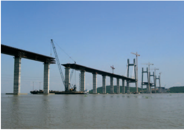
Figure 1: The second bridge over the Orinoco River under construction.
