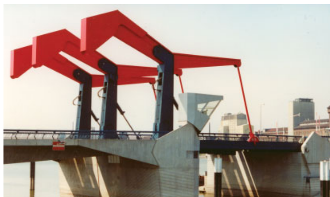
Bild 7. Diffené-Brücke in Mannheim [9] Fig. 7. Diffené bridge at Mannheim [9]
