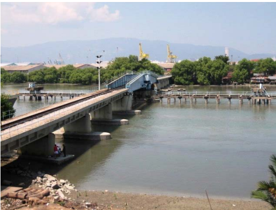
Fig.1: Existing river bridge
